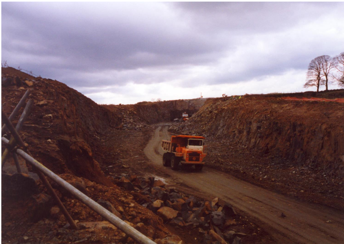
Fig. Q.4 Motorway construction operations in hard rock overlain by a 2 m stratum of glacial clay.
